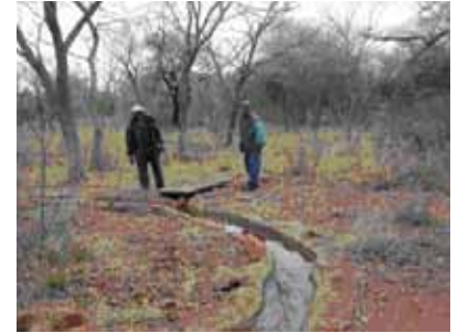
Solar powered water point
